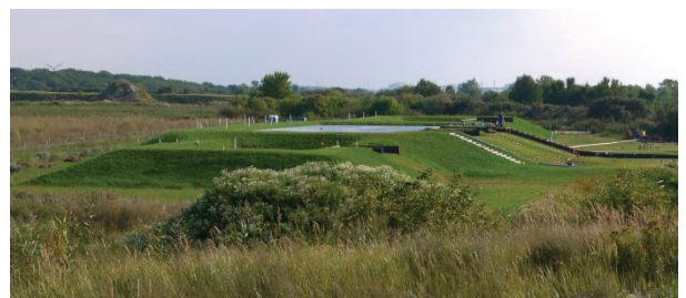
Fig. 1. Rostock research dike with filled polder 2, north view
