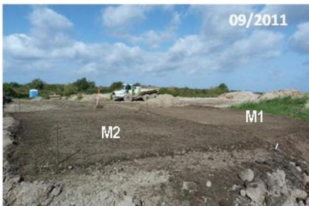
**Fig 9.** Prepared compaction testing field
