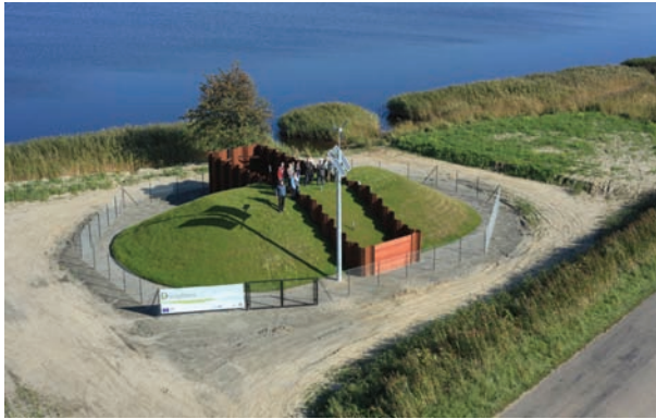
Fig 1. The prototype dike near Gdansk, constructed from composite soil
