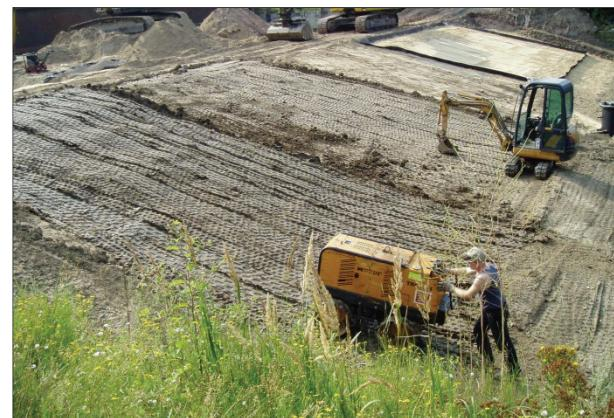
**Fig 2.** Construction of the test fields in August 2004: Compaction of layers of marsh sediment
