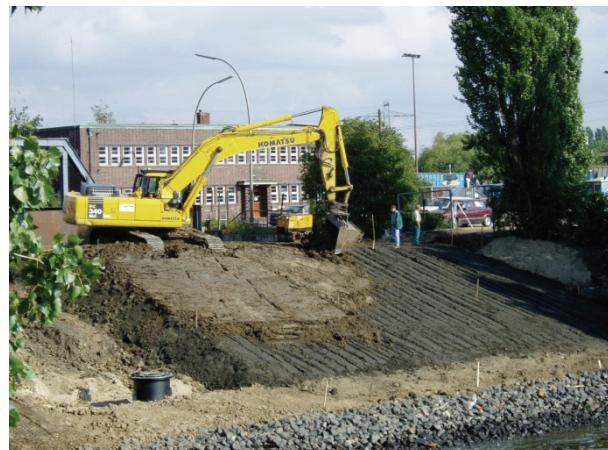
**Fig 1.** Construction of the test fields in August 2004: Construction of the cover layer (marsh sediment) on layers of processed dredged material. On the left: collection chamber
