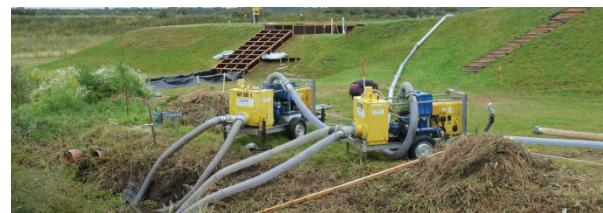
**Fig. 3.** Two pumps deliver water into the polders
