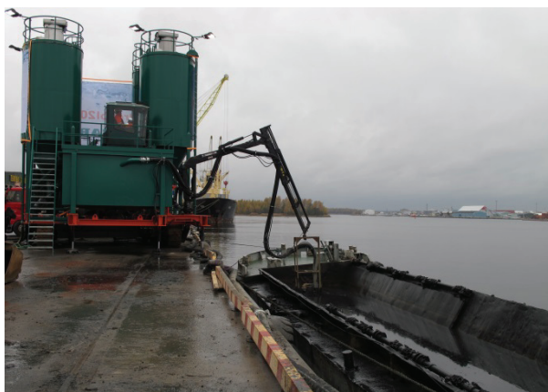
Fig 5. The dredged sediments are pumped into the process stabilization equipment
