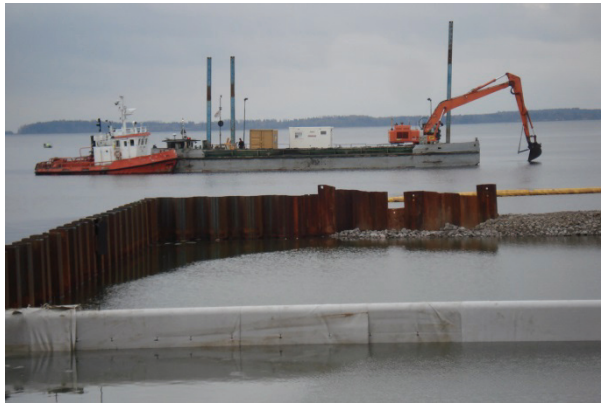
Fig 4. The basins to be filled with s/s-treated sediments
