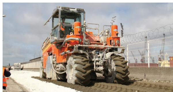
**Fig 7.** Treatment of the sediments on the Freycinet road
