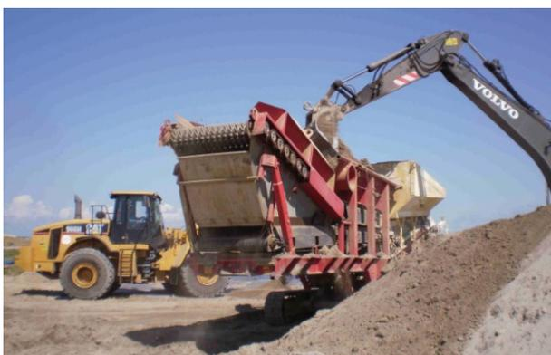
**Fig 9.** On site pre-treatment of lagooned sediments with the CSA additive.
