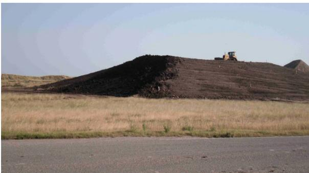
Fig 2. Sediment dike under construction
