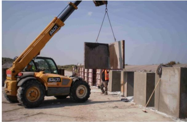
**Fig 10.** Demoulding of the blocs on site
