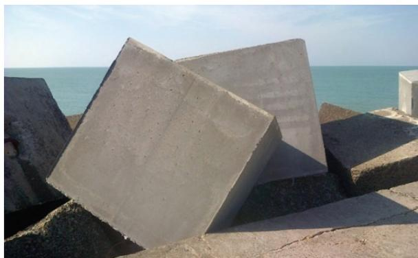
**Fig 11.** First concrete blocks containing contaminated sediments on the Digue des Huttes at Dunkirk (Sept. 2013)
