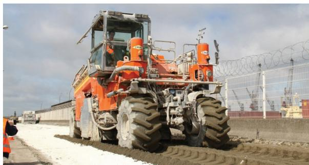
**Fig 7.** Treatment of the sediments on the Freycinet road
