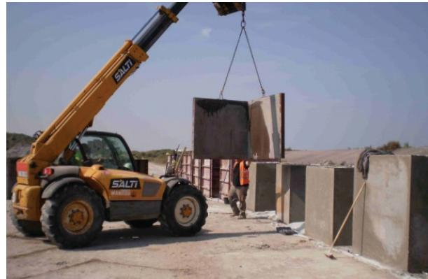
**Fig 10.** Demoulding of the blocs on site
