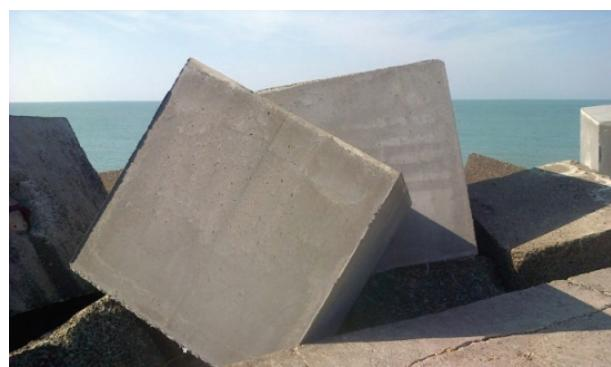
**Fig 11.** First concrete blocks containing contaminated sediments on the Digue des Huttés at Dunkirk (Sept. 2013)
