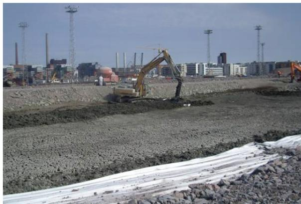
**Fig 16.** Stabilisation work in basin 2, 2011 (in the front right corner - stabilisation machine running; at the back - loading embankment and geotextile)
