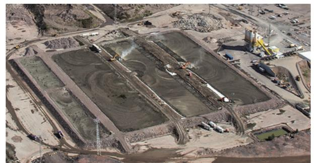
Fig 15. The aerial photos of the stabilisation basins. Stabilisation process on-going (by the City of Helsinki).
