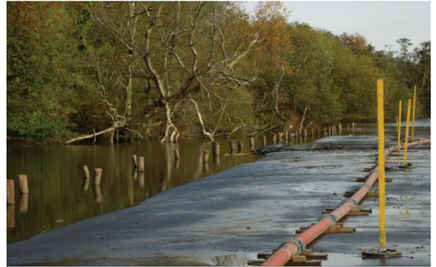
**Fig 6.** Gauging rods placed into the geotextile tubes.
