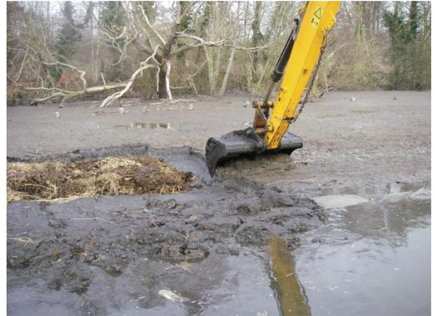
**Fig 10.** Scraped vegetation placed on the geotextile tubes, March 2013.
