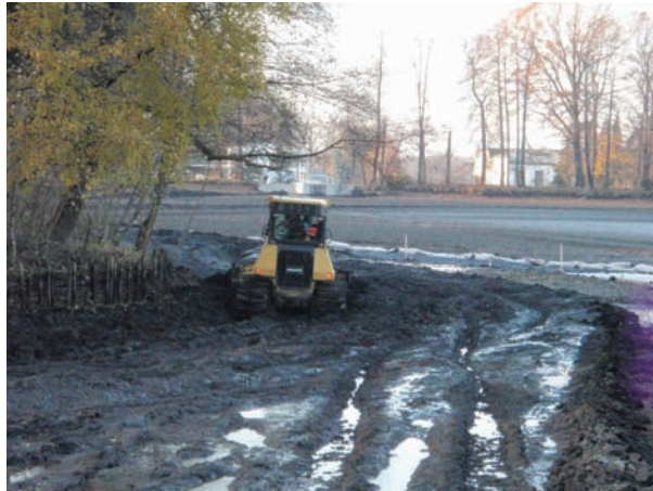
Fig 8. Mass removal of sludge with bulldozer
