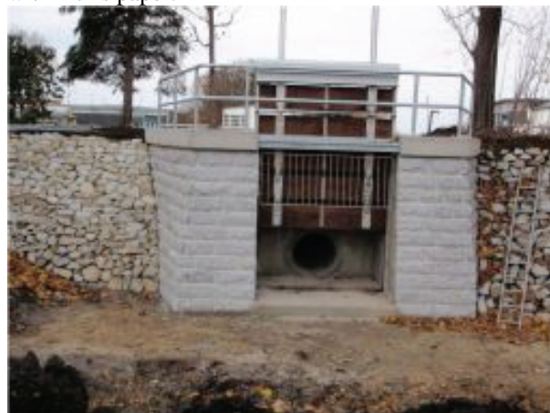
Fig 4. New Outlet construction
