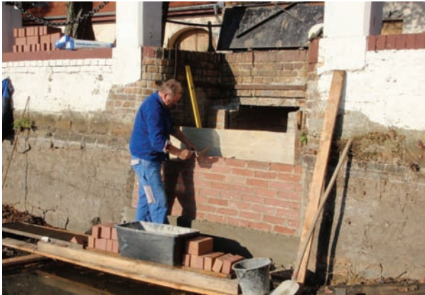
Fig 5. Shutting down the old outlet
