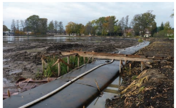
Fig 13. Tubes during filling process and new fishing spots still under construction
