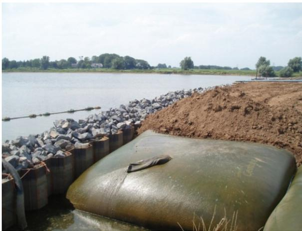
Fig 3. Covering tubes after consolidation of the infill
