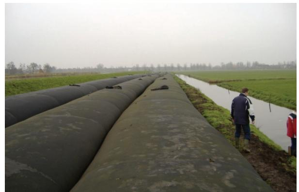
**Fig 5.** Tubes filled on the dike
