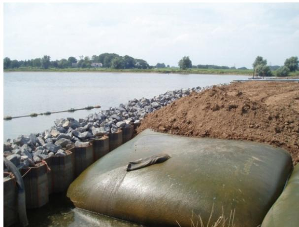
**Fig 3.** Covering tubes after consolidation of the infill
