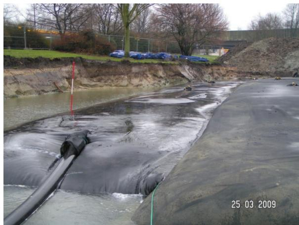
**Fig 7.** Tubes, at filling and dewatering at site
