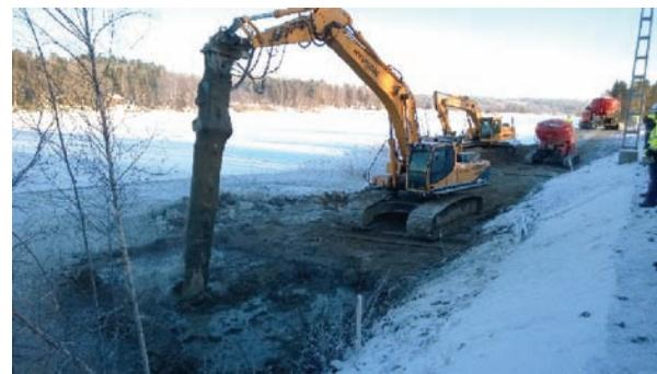
**Fig 9.** Railway embankment support by mass stabilising. Stabilisation work in progress at -20°C temperature.
