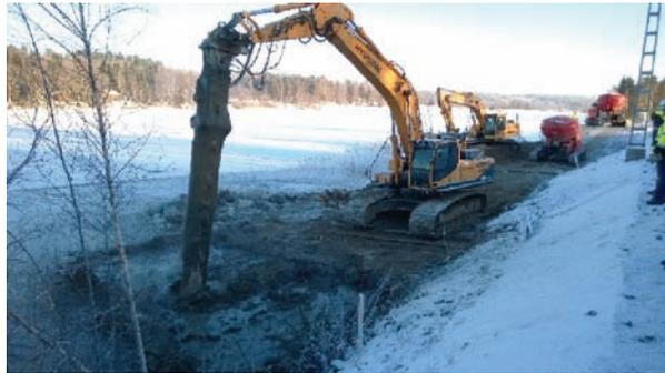
**Fig 9.** Railway embankment support by mass stabilising. Stabilisation work in progress at -20°C temperature.
