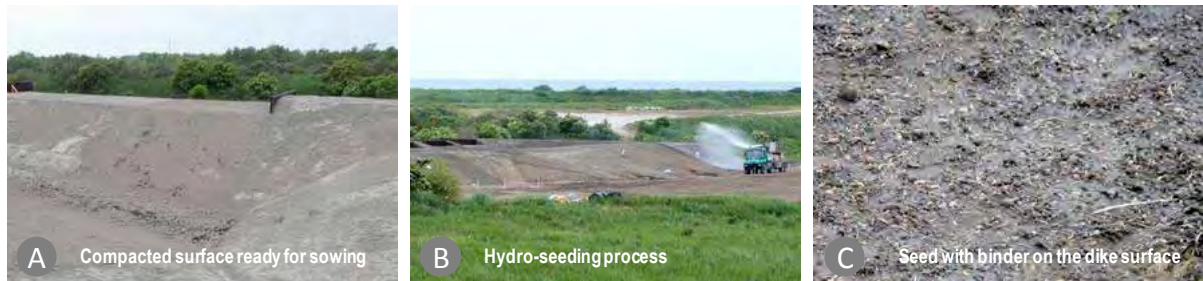
Figure 11. Preparation and sowing at the test dike
