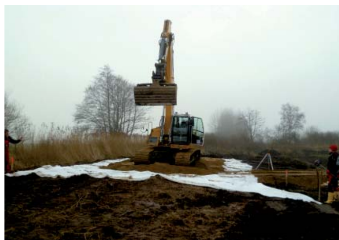
Fig. 3: Constructing the dike core on a woven reinforcement geotextile
