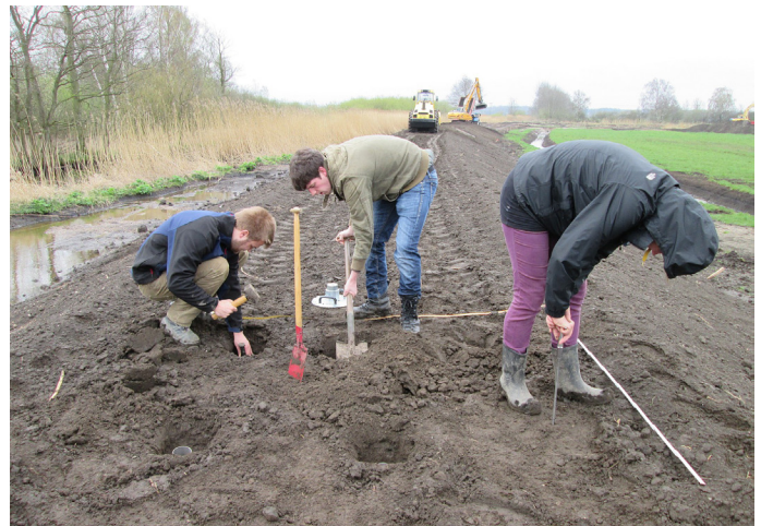
Fig. 5: Construction of the pilot dike and quality control by students
