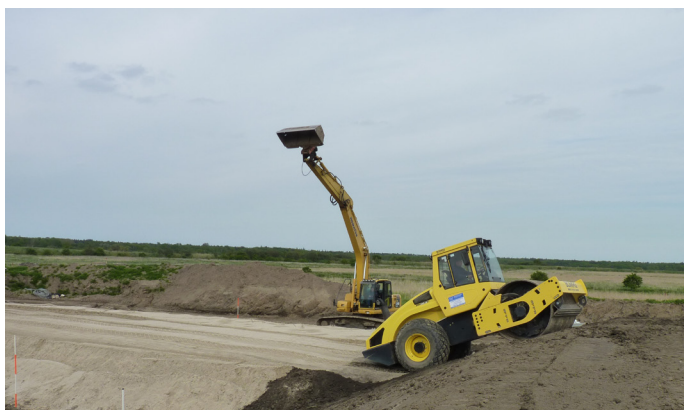
Fig. 3: Construction of the Rostock research dike
