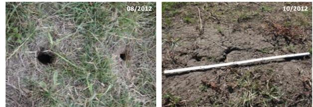
Figure All.62. Activity of voles (l) and crack on the research dike (r)
