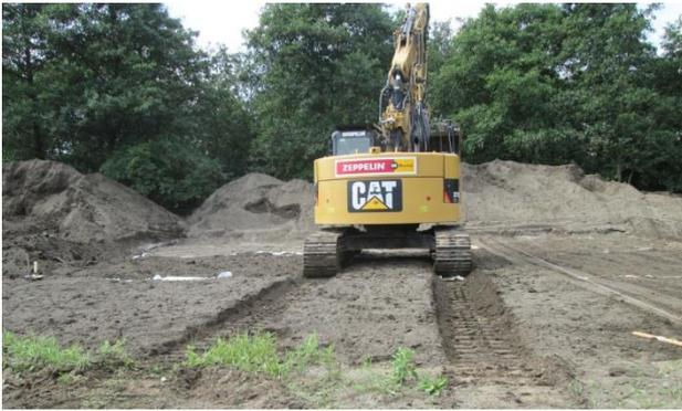
Figure All.136. Compaction with the excavator tracks only
