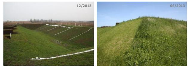
Figure All.61. Turf development at the test dike; polder 2 in 2012 (l), polder 1 in 2013 freshly mowed (r)
