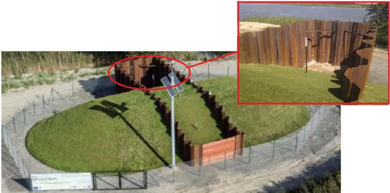
Figure All.84. Polish research dike with sheet pile basin
