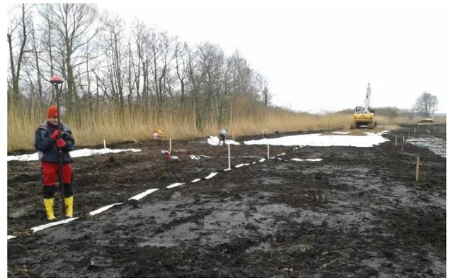
Figure All.133. Construction of the dike core with geosynthetic reinforcement and wire placement underneath the dike 12-2013
