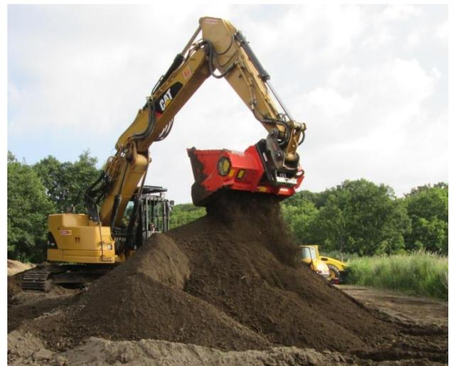
Figure All.139. Soil homogenisation with screener crusher
