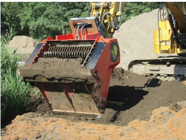
Figure All.141. Mixing of fibres and DM with the screener bucket
