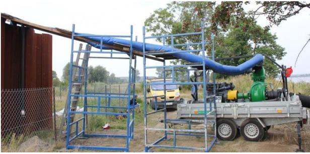
Figure All.94. The pump delivers water into the sheet pile basin
