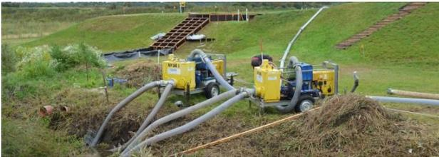
Figure All.13. Two pumps deliver water into the polders
