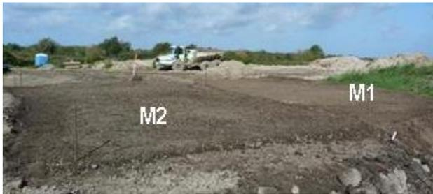
Figure All.51. Prepared compaction testing field
