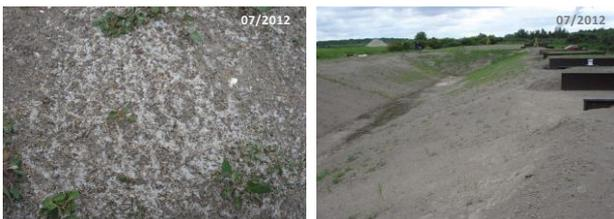
Figure All.60. Surface of test dike two weeks after hydro-seeding; decomposed binder (l), beginning saltbush growth (r)
