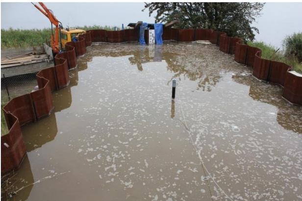
Figure All.95. Filled sheet pile basin
