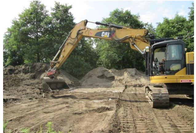
Figure All.135. Compaction with the excavator shovel only
