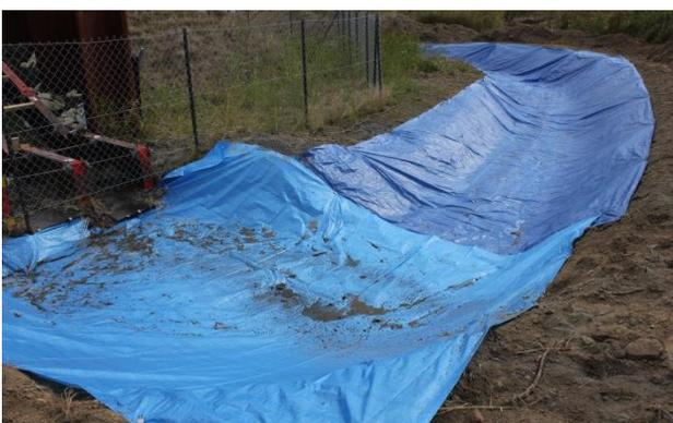
Figure All.97. Runoff channel to lead the water back to the Vistula
