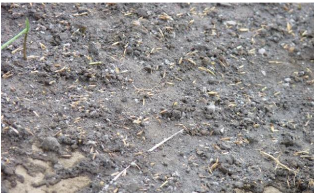
Figure A1.16. Hydro-seeding on a compacted surface of the DredgDikes research dike in Rostock
