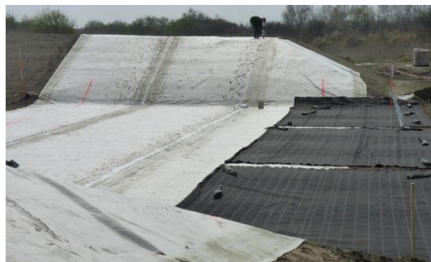
Figure A1.14. GCL installation at the Rostock research dike
