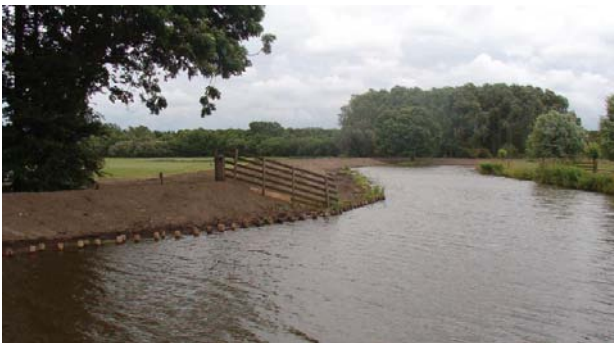
Figure 2.19. Placement of dredged material on banks of waterways in the Netherlands [20]
