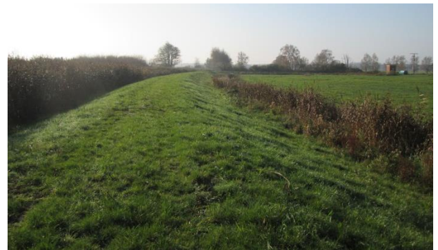
Figure 1.4. DredgDikes pilot dike construction east of Rostock
