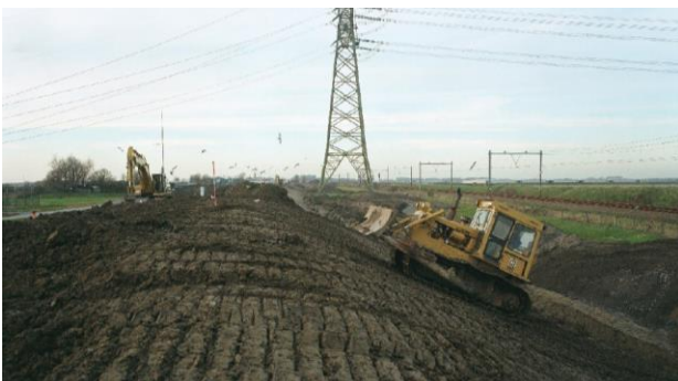
Figure 2.20. Dike construction at Hoek van Holland [20]
