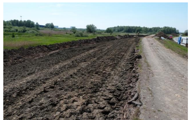
Figure 2.17. Dike reconstruction in Bremen with slightly contaminated dredged material (Z2 + TBT), DM placement summer 2014.
