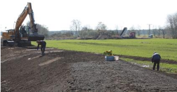
Figure 5.13. Seeding and raking in by hand on the DredgDikes pilot dike
