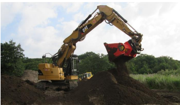
Figure 5.3. Homogenisation of DM with screener fixed to an excavator
