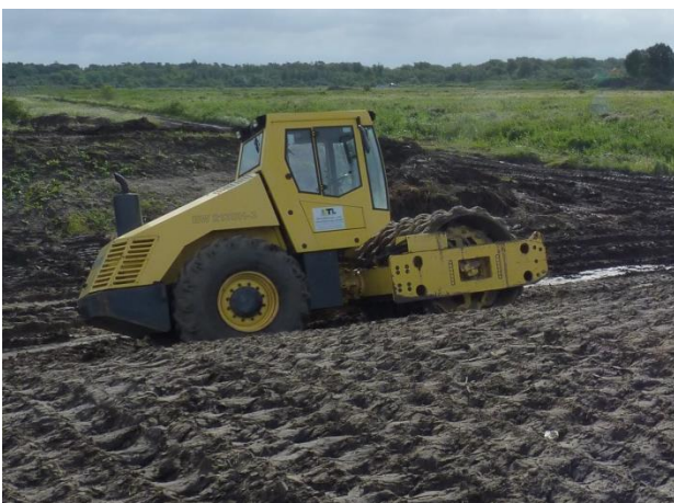
Figure 5.5. DM compaction with a sheep's foot roller compactor
