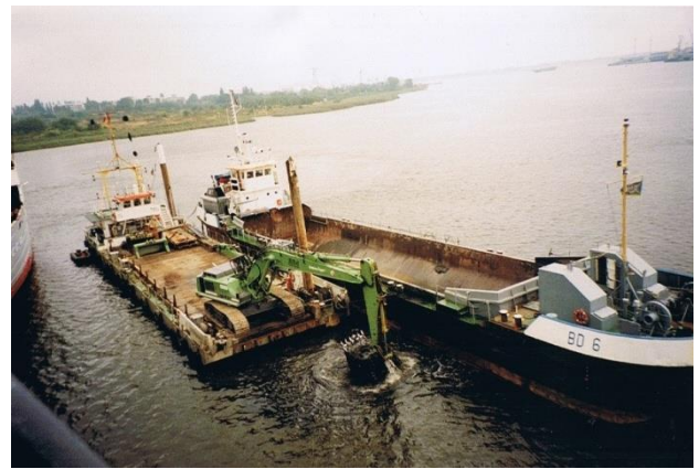
Figure 2.1. Dredging works at the Warnow tunnel in Rostock, dredging of fine grained organic silt
