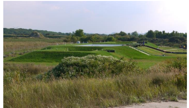
Figure 1.2. DredgDikes research dike in Rostock
