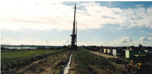
Figure 5.9. Vertical barrier construction (courtesy Moebius Polska)
