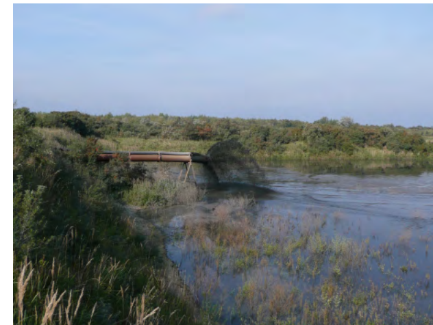
Dredged material pumped onto a spoil field
