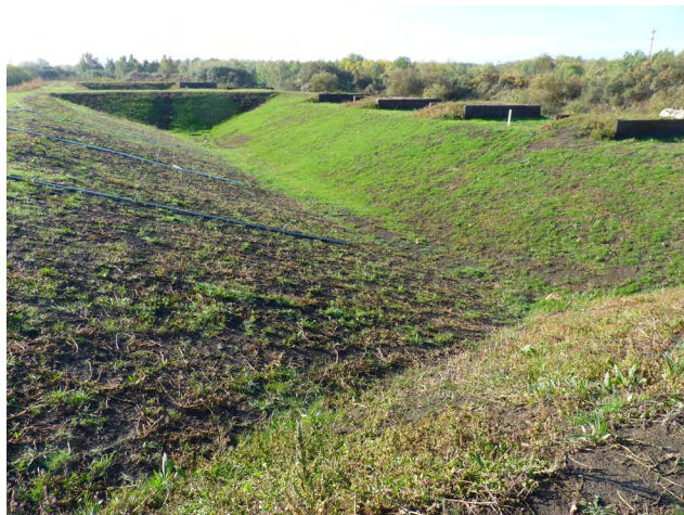
Section two of the Rostock test dike
